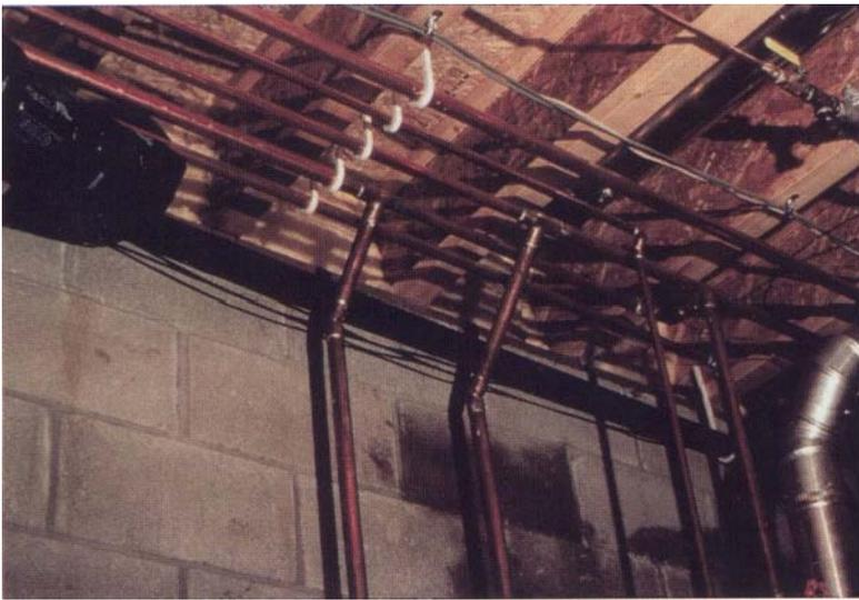
Copper tubing installed in a typical water distribution system. Under normal circumstances, installed copper tubing can last the life of a building. Photo courtesy of the Copper Development Association, New York, New York.
